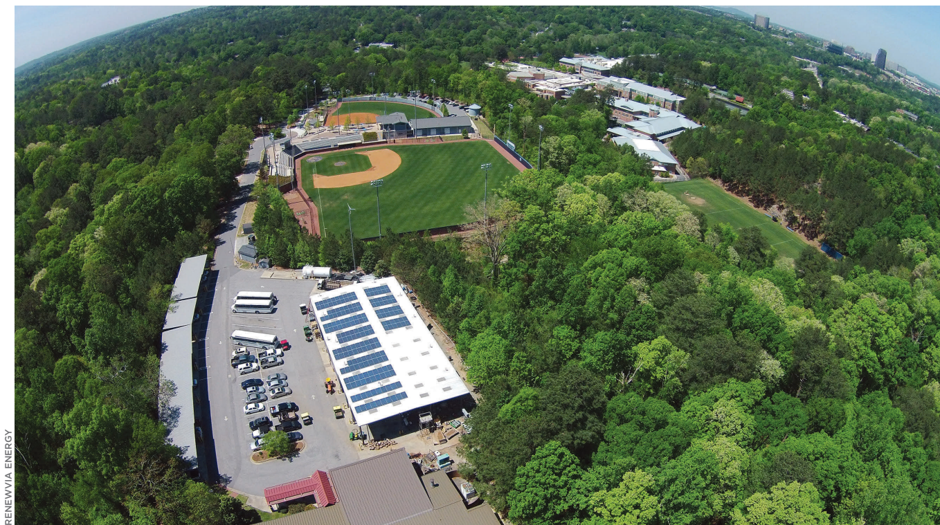
Figure 1. Solar rooftop arrays installed on The Lovett School in Atlanta, Georgia.
