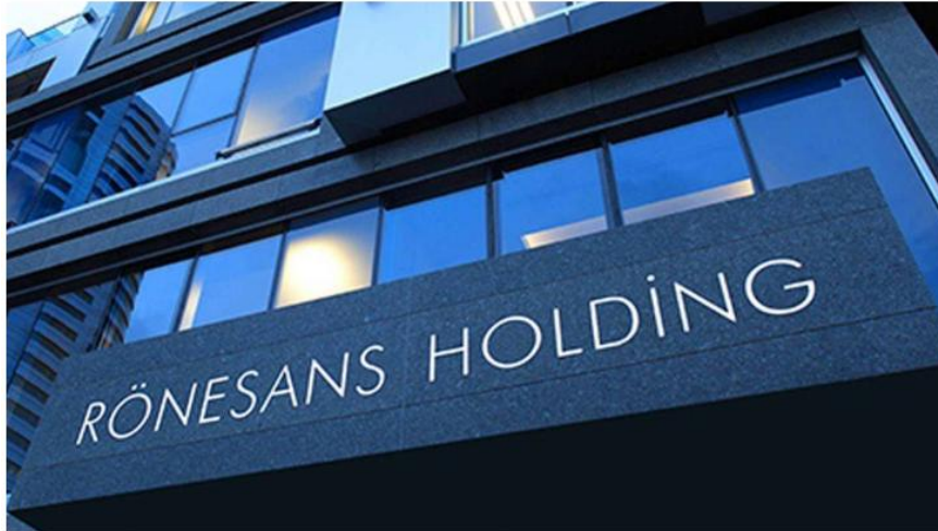
Fig 15: Turkish Holding Company Renaissance is based in Ankara and its main activities are construction and real estate investment.
